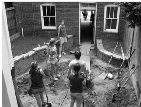
WQW workers removing 18 inches of topsoil
