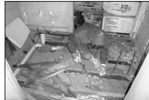
WQW Workcamper doing renovation project in home of Capitol Hill neighbor
